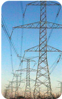
Figure 1 Transmission lines, supported by tall metal towers, carry high voltage electricity over long distances.
